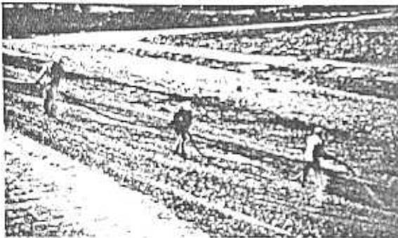
(e) Spraying water on trimmed slope
