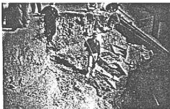
(1-a) Severe collapse of fill material under concrete slab of an irrigation canal
